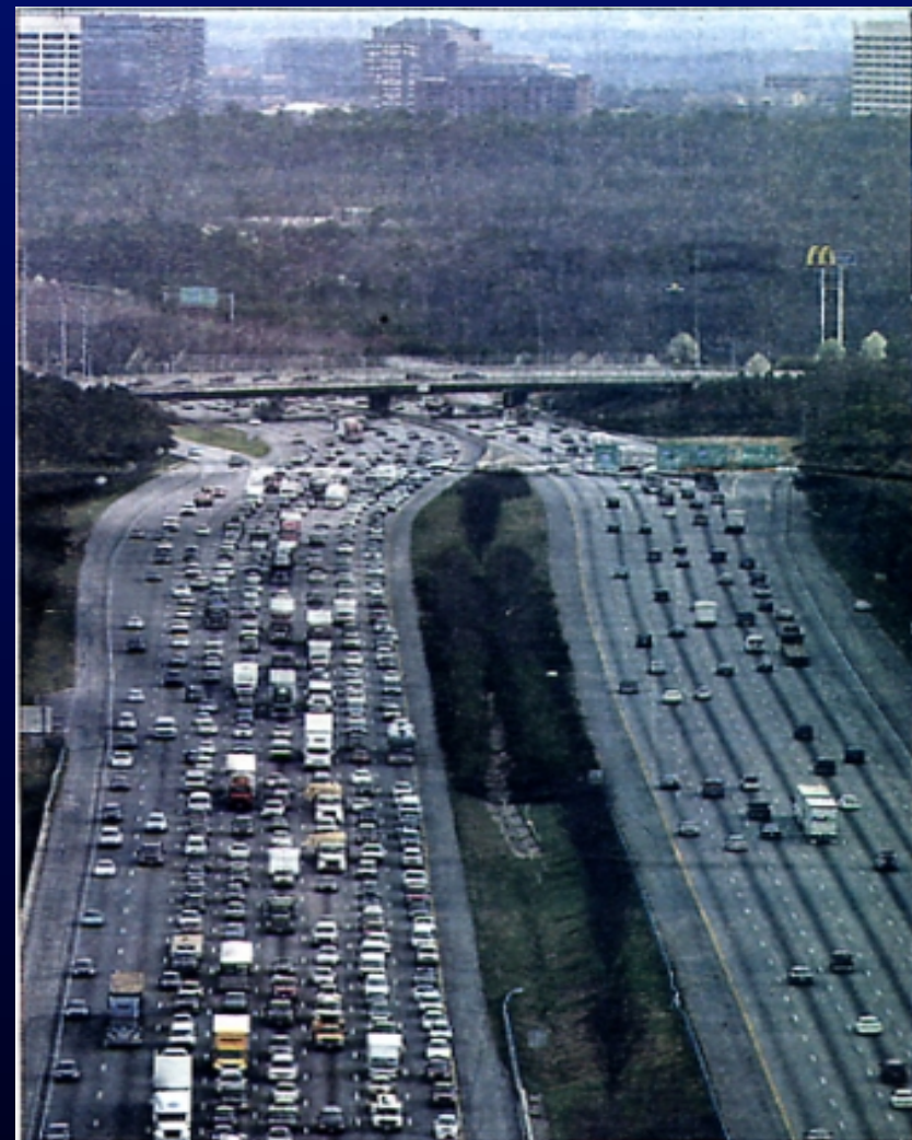
Traffic heads north on I-75, just north of I-285, on Thursday. A proposal for the interstate is enough to make a road builder weep with joy, and make others wonder whether it's overkill. LOUIE FAVORITE / Staff
